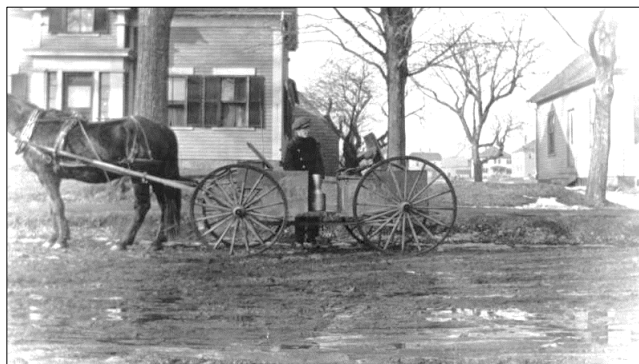
Earl P. Sawtelle delivering milk, possibly on Church Street about 1900. This was in the era before home delivery by major dairies, and long before the end of home deliveries!
