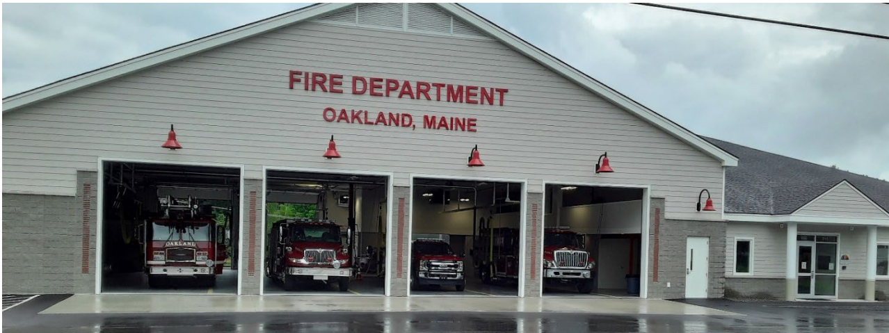
Oakland's new Fire Department, 2021 (Author's photo)
