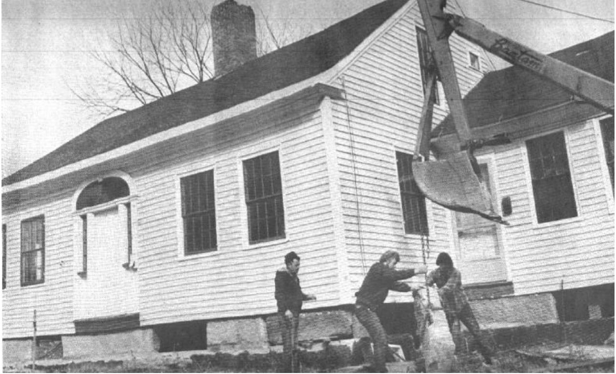
Moving the Macartney House (photo courtesy OAHS).
