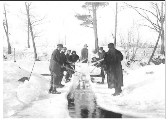
Cutting Ice, on the lake. The ice was cut with large horse-drawn blades, then floated along the channels thus produced, all the way to the ice houses
