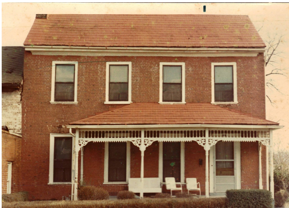
Either One Richardson's House, 108 South First St, before renovation
