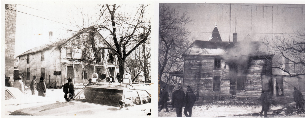
(Photos of fire at apartment house, 9 Jan 1971)
