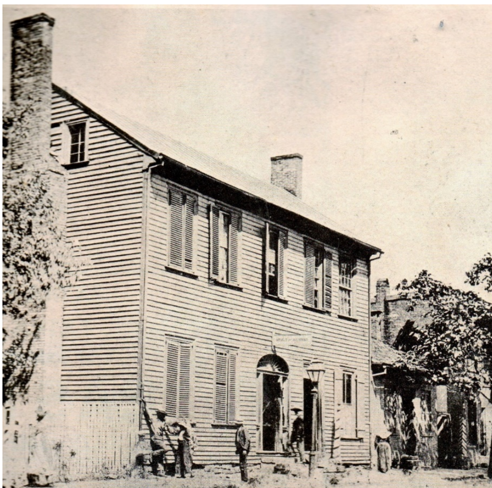
The McDowell House prior to renovation, 1939
